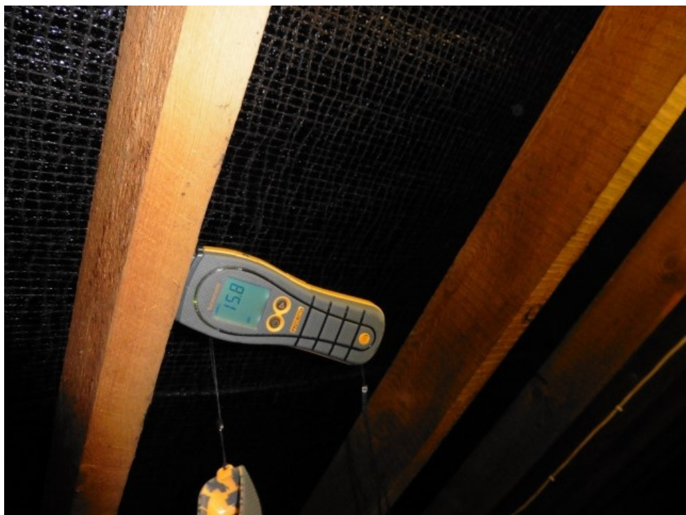
Normal moisture reading in roof timber
