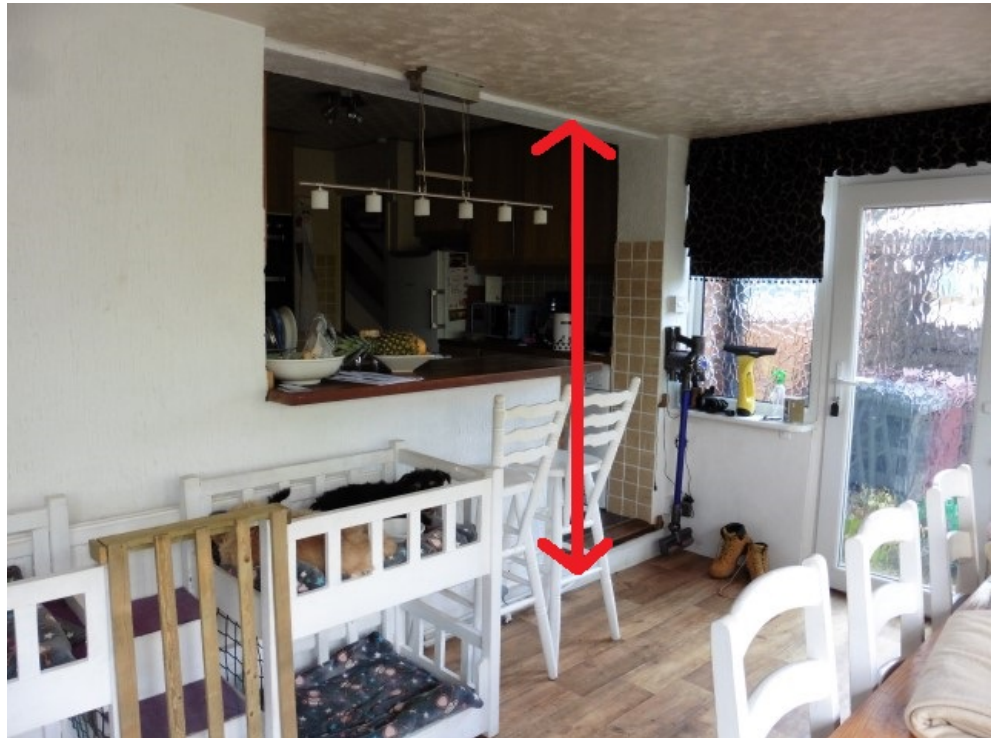
Wall partially removed between the kitchen and sun room
