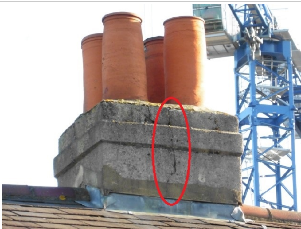
Central stack viewed from the front
