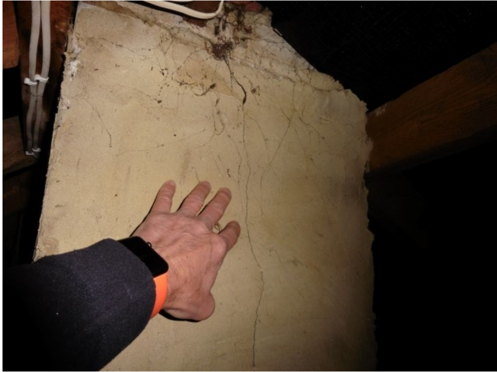
Light cracking of the right side chimney breast in the roof space
