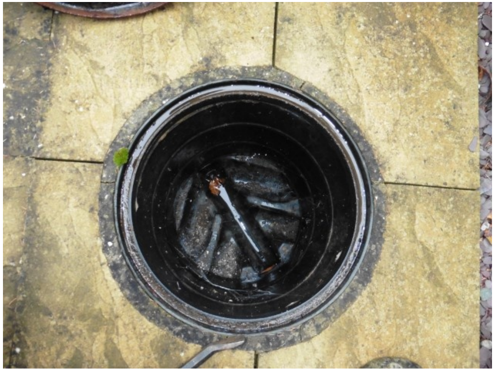
Inspection chamber to the front
