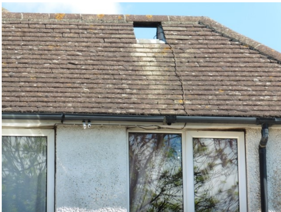
Rear roof pitch
