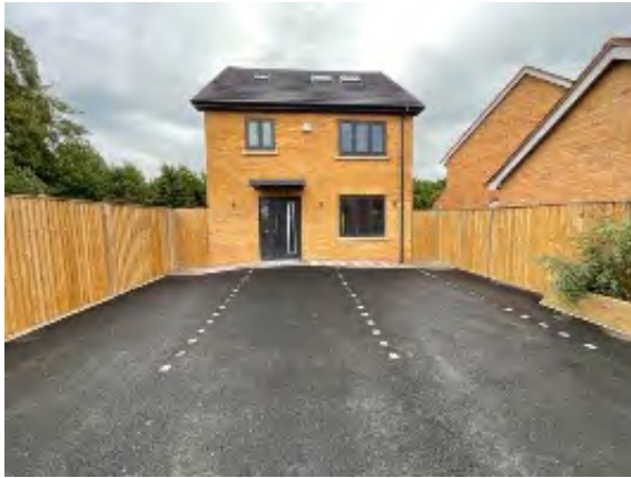
3. Front parking area
